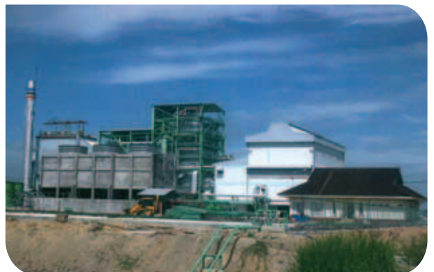
:: 9.9MW EFB Power Plant Surathani, Thailand 2,500 m 3 /hr.
