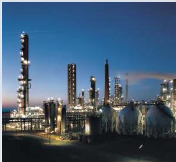
In the petrochemical industry, it is the LR system that provides reliable and fault-free power supply.
